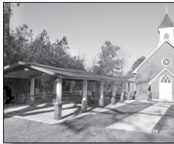
New pavillion built in 2011
